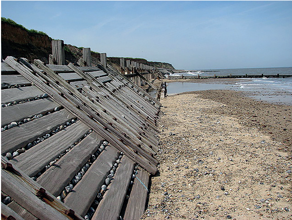
Fig. 1.7 for Question 1 Revetments
