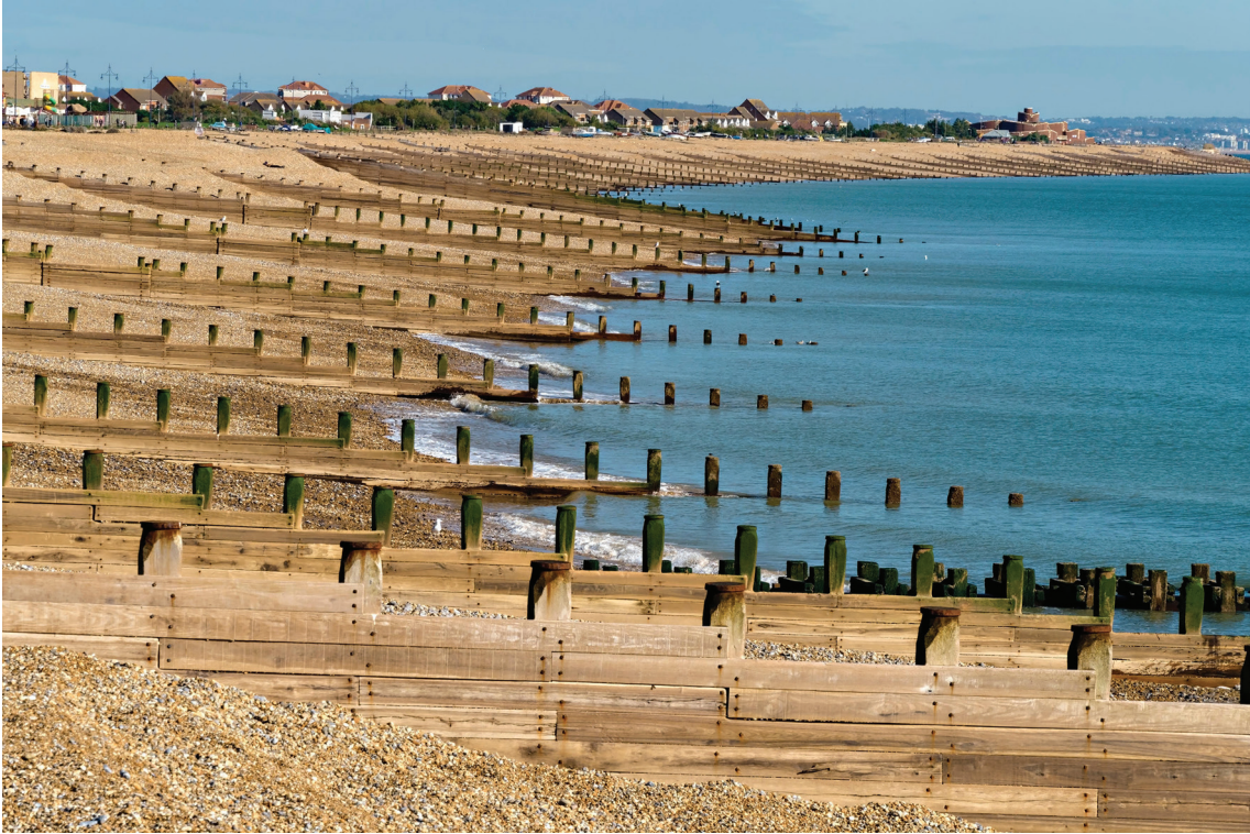
Fig. 1.5 for Question 1 Groynes
